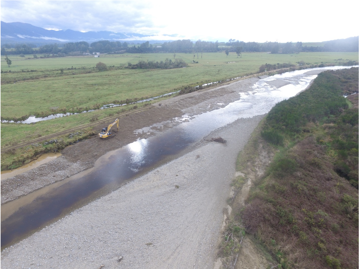
Nelson Creek stopbank repair, 1km above the State Highway Bridge.
