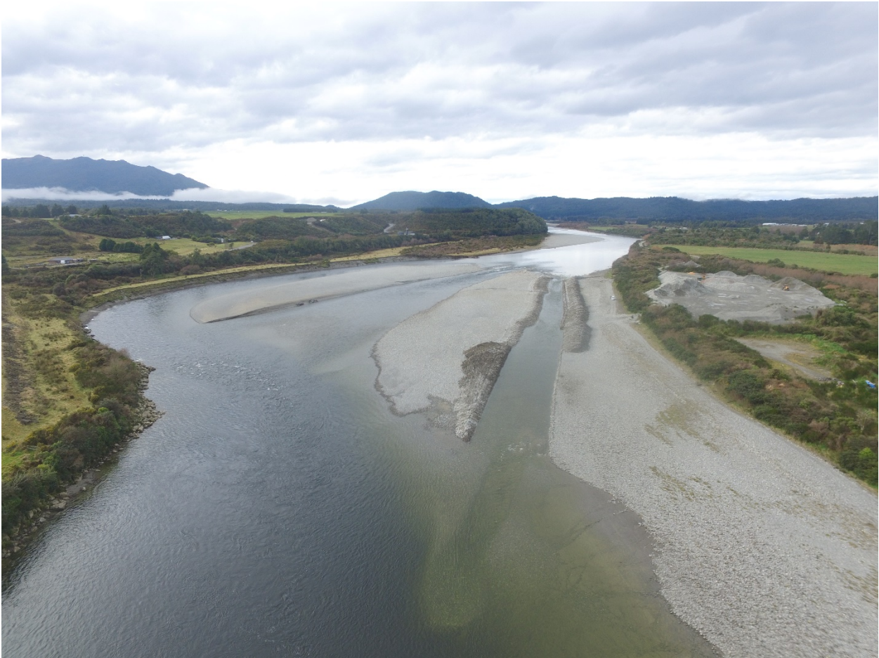
Diversion cut on the Grey River at Coal Creek, looking upstream
